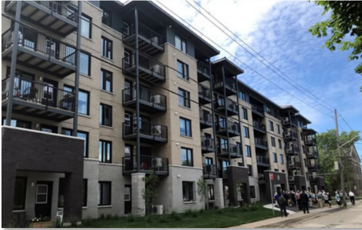
Wall Street Village - Brockville
