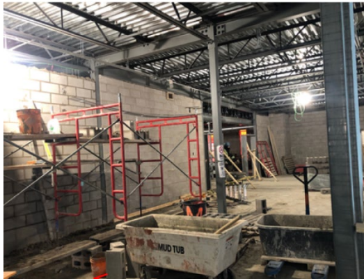
Interior block clean Linen room
