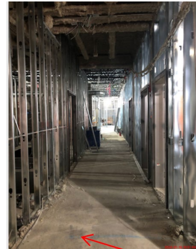
Ground floor corridor looking East
