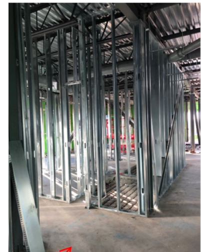
Mockup suite framing
