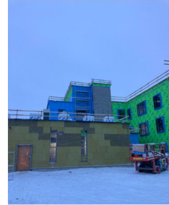
Insulation & vapour barrier works
