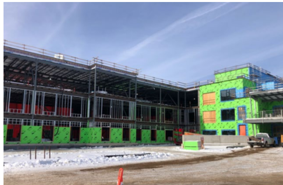
South-East floor exterior wall framing
