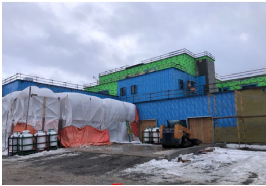
Masonry hoarding & temporary heating
