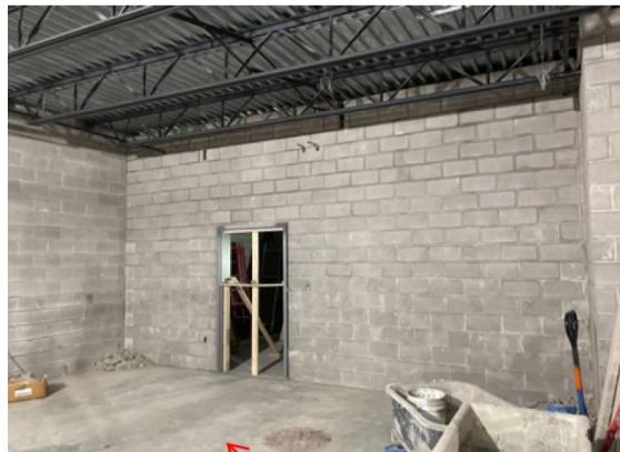
Block works within Refrigerated Garbage/Recycling room
