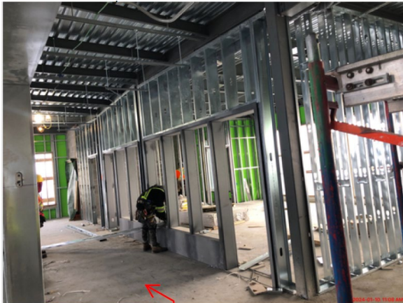
2 nd floor board room framed
