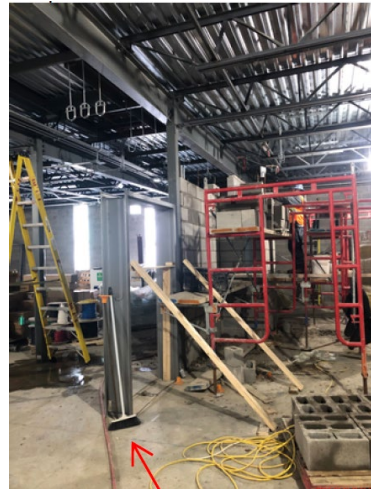
Interior block works at refrigerated rooms
