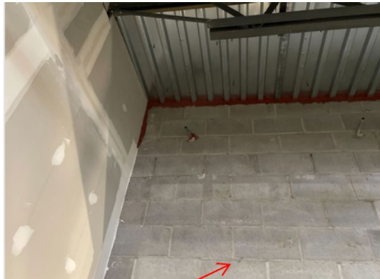
Fire caulking works at Penthouse
