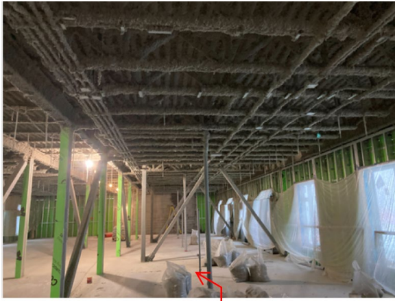
Ground floor North wing fire spray activities
