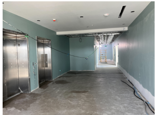
T-Bar nearing completion 3rd Floor Core Elevator Corridor
