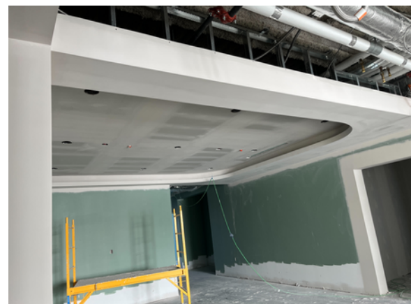
2nd Floor Core Elevator Vestibule
