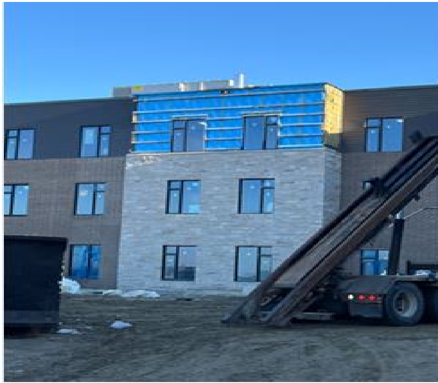
Stone Works Complete Rear of Building Bump Out/Siding Preparation
