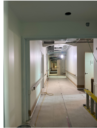
NW Corridor Railing
