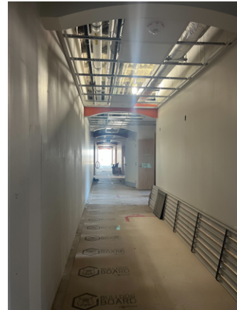
SW Ground Floor Private Suite Corridor Doors/Flooring
