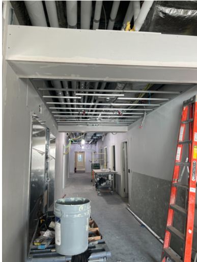
Ground Floor Core Elevator Vestibule Ceiling Progress
