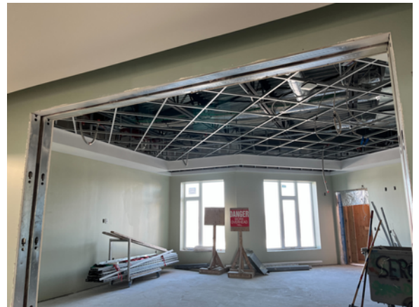
SW 3rd Floor Dining Rooms T-Bar Complete
