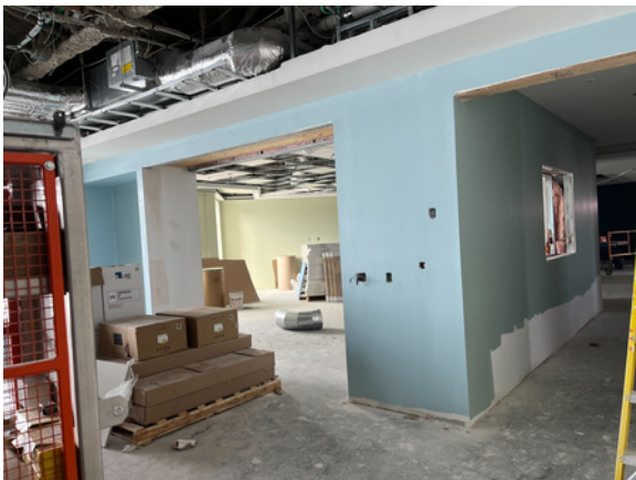
2nd Floor NW Dininf Room Paint
