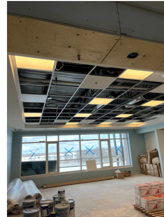
3rd Floor NW Dining Room Ceiling
