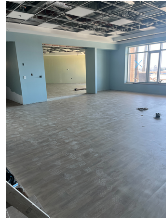
SW 3rd Floor Dining Room Flooring ...
