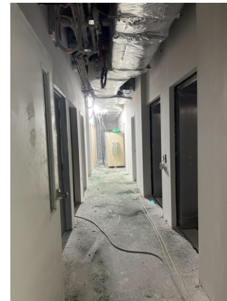
Corridor 0208 Ready for Paint
