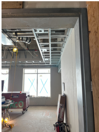
Ground Floor Meeting Room Bulkhead
