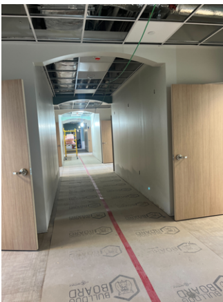
Ground Floor SW Semi Private Corridor Doors and Flooring
