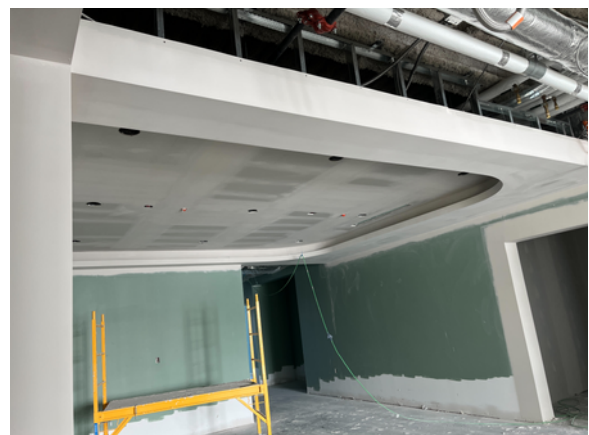
2nd Floor Core Elevator Vestibule Bulkhead Finishing Progress
