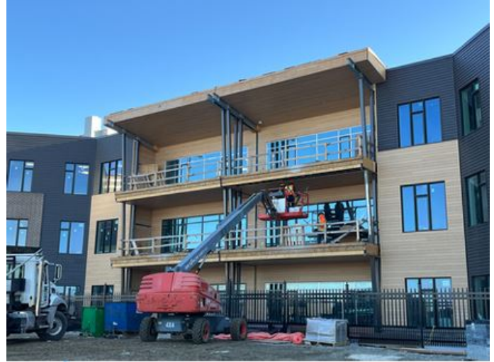
Rear Canopy Siding Nearing Completion
