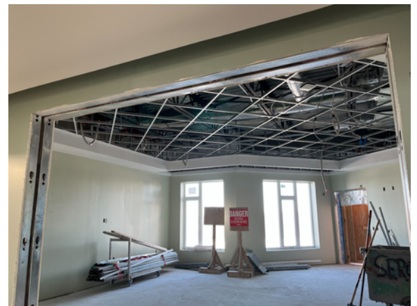
SW 3rd Floor Dining Rooms T-Bar Complete
