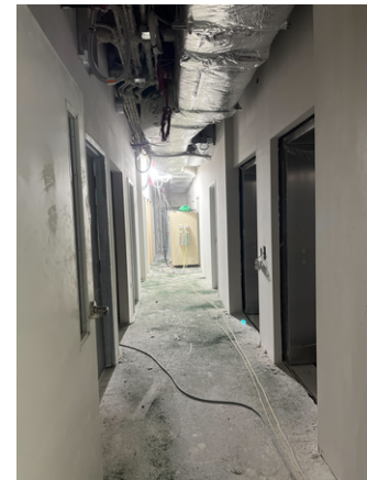
Corridor 0208 Ready for Paint
