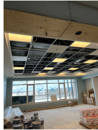
3rd Floor NW Dining Room Ceiling Progress - Lighting
