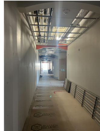
SW Ground Floor Private Suite Corridor Doors/Flooring
