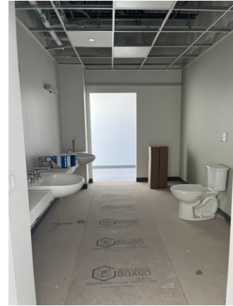
SW 3rd Floor Semi Private Suite Sinks/ Toilets Installed
