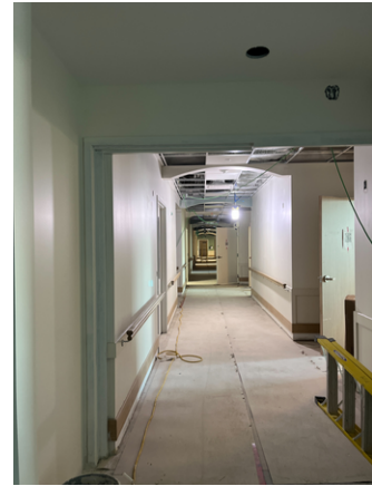
NW Corridor Railing
