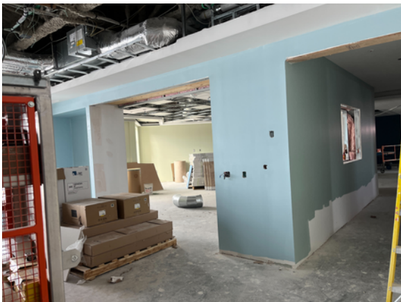
2nd Floor NW Dining Room Paint Progress
