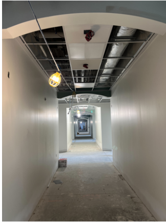
SW 3rd Floor Corridor Lighting/Device Installs
