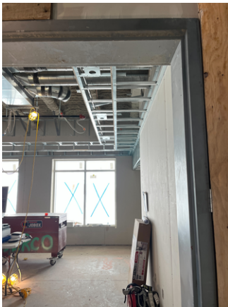
Ground Floor Meeting Room Bulkhead
