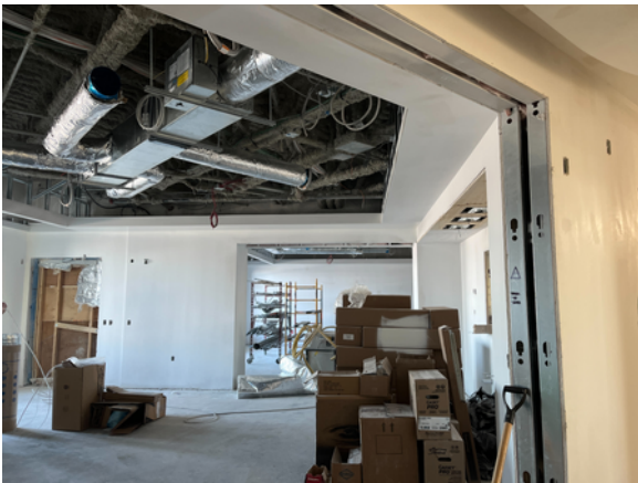
SW 2nd Floor Dining Rooms Ready for
