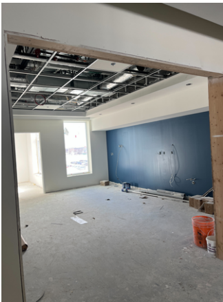
SW 3rd Floor Common Area Room Finishing Progress
